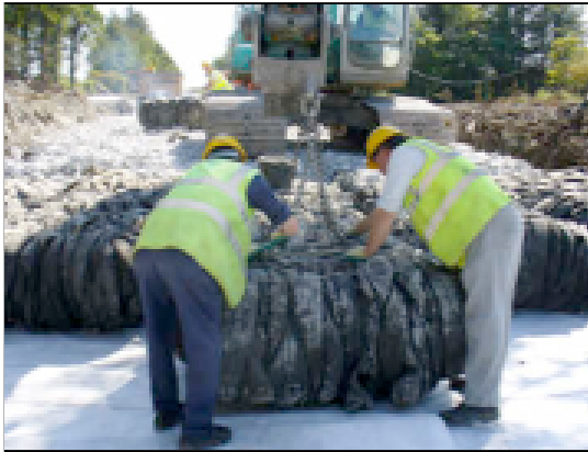
Replacement Road Construction, Mounbellaw, Co Galway.
